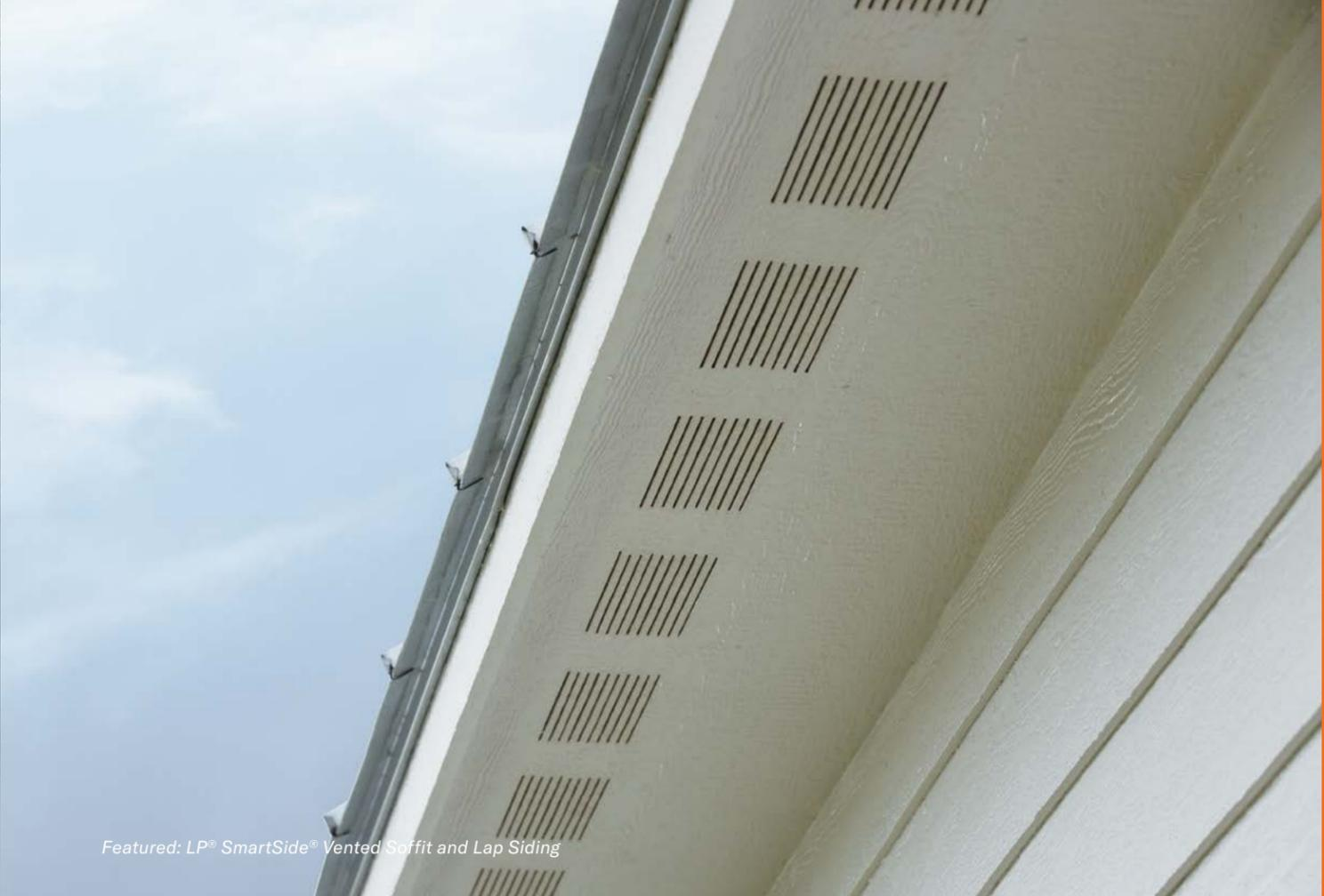
Featured: LP® SmartSide® Vented Soffit and Lap Siding
