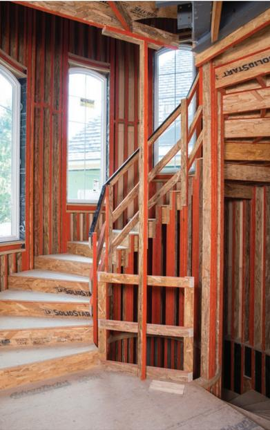
LP Building Products in previous builds, Ennis chose to use LP SolidStart LSL and LP® TechShield® Radiant Barrier Sheathing. For the pool wing, Ennis and the homeowner selected LP products due to their quality, consistency, and cost efficiency compared to concrete masonry units (CMUs) that the architect had originally specified.
