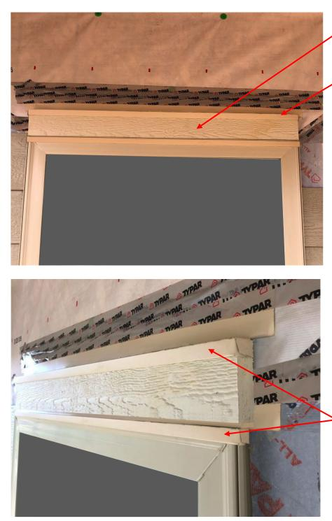
Properly install 5/4 trim over window and maintain min. 3/8" clearance above Z-flashing (touch-up cut ends of trim)
