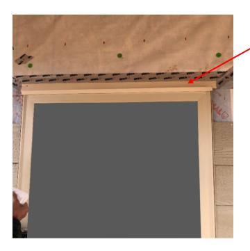
Properly install sloped Z-flashing above window (add flashing/WRB tape as needed)
