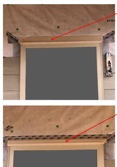
Properly install sloped Z-flashing above window
