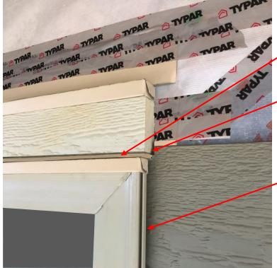
Maintain minimum 3/8" clearance above Z-flashing
