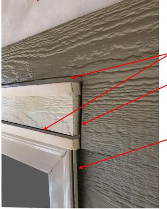
Maintain minimum 3/8" clearance above Z-flashing
