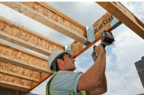
That’s because the Simply Better 225i has a more consistent moisture content that makes the product less prone to such issues as twisting, warping and shrinking. The wider flange also offers an easier nailing surface and increased stability for enhanced floor performance.
