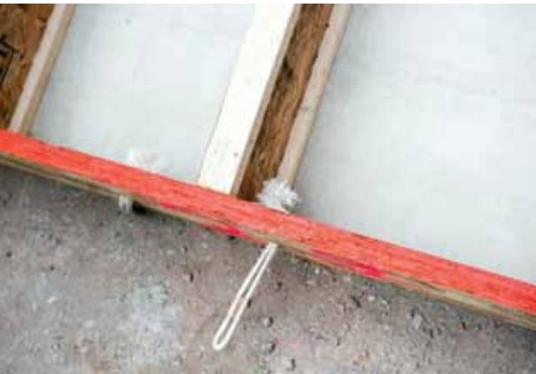
Plus, LP SolidStart I-Joists offer greater straightness, depth and length than traditional timber, and they are significantly lighter depth-for-depth. LP SolidStart LSL was used on the top and bottom of the frames to provide additional strength in the plates where a positive connection is needed most.
