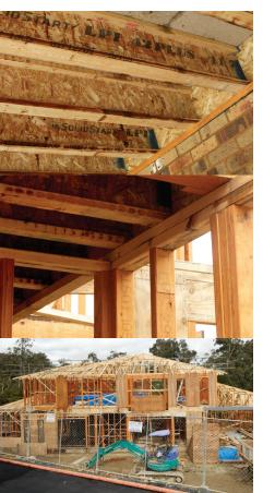
He said the home has a lot of load bearing walls, so the durability and stability offered by LP SolidStart Engineered Wood Products appealed to him. He added that LP SolidStart LVL is superior to other timber products, which are hard to find at longer lengths.
