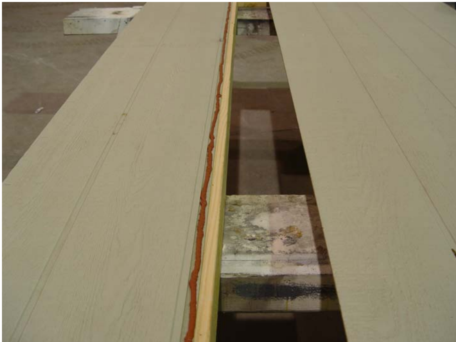
View of vertical joint with fire caulk application
