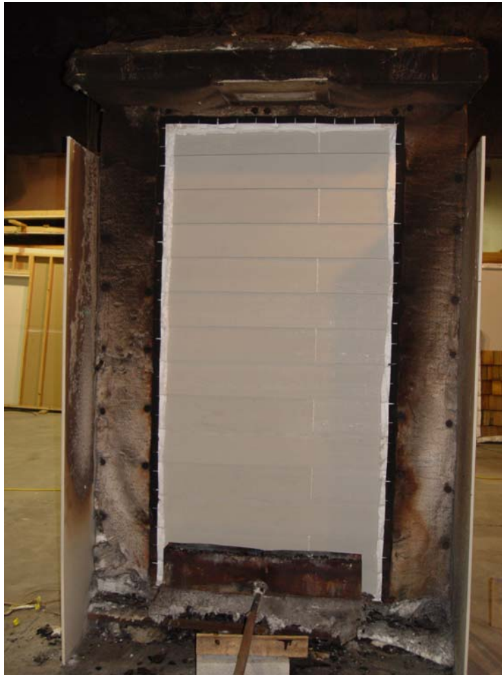
Series 5, 1/2" LP Smartside® Foundation Series exterior lap siding – wet process fiber back-bone, 8" wide, 1" overlap, 16" face nailing, applied over 5/8" type X gypsum wallboard (reference WFCi P/N 07058, Tests 10, 11 & 12)
