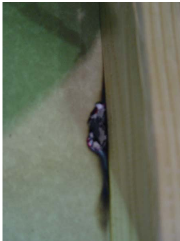
Series 3, Test 3, Nonfire side at test termination (70 minutes)
