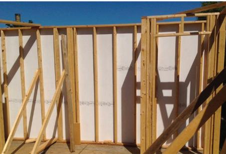
Allen chose to have LP FlameBlock sheathing installed as a part of the code-compliant U350 assembly in hopes that it would simplify the assembly process for his volunteers. He also wanted to avoid any safety hazards that a traditional shaft assembly wall may pose due to the complexity of the construction.
