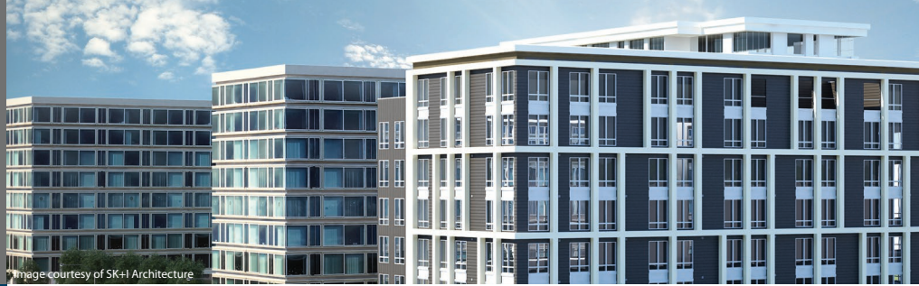
Image courtesy of SK+I Architecture
