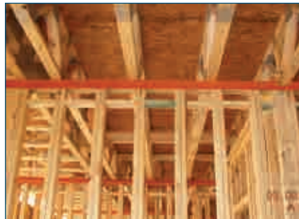
LSL top wall plates
