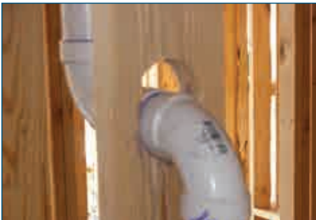
Example of allowance for building shrinkage
