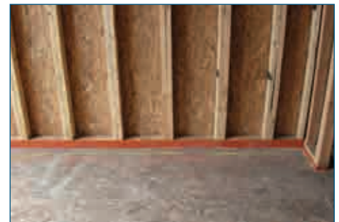
LSL bottom wall plates
