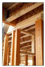
recommended screwing or nailing attachment for ceiling plasterboard (or high temperature wall or bracing areas). For floors use the recommended screwing (or nailing) attachment for flooring. Glue will not adequately stick to the LP SolidStart LVL studs and joists with SiteCote and/ or wax edge seal.
