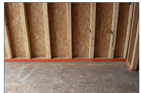
LSL bottom wall plates
