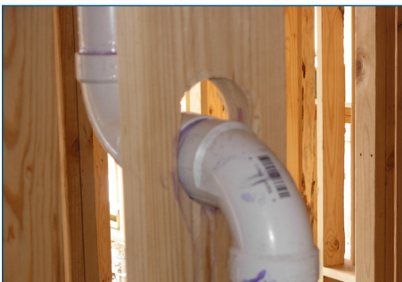
Example of allowance for building shrinkage
